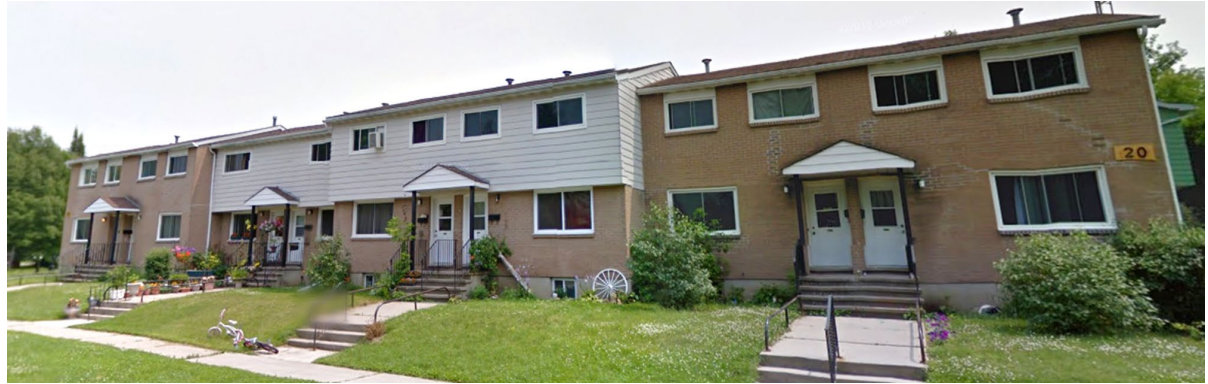
LCHC: Robinson Street, Perth
