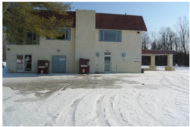
Image 5: View of the north elevation of the Clubhouse.
