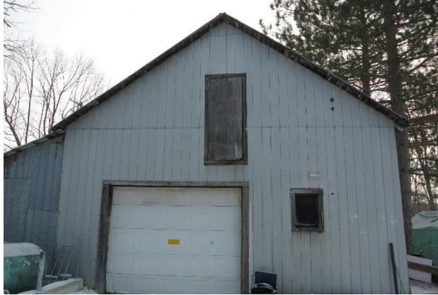
Image 10: View of the west elevation of the one-and-a-half storey accessory building.
