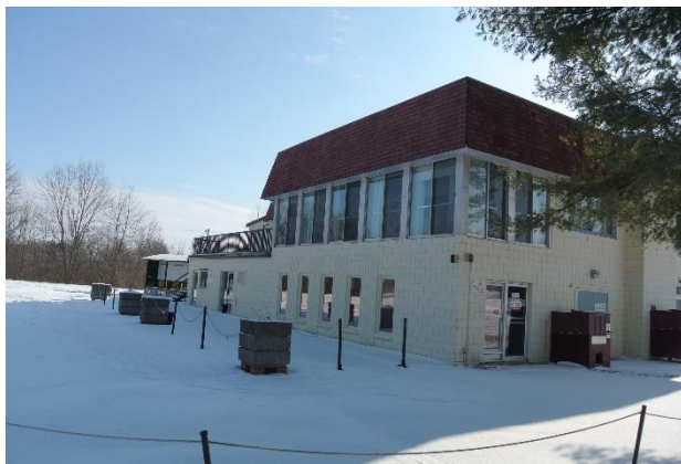
Image 4: View of the east elevation of the Clubhouse.
