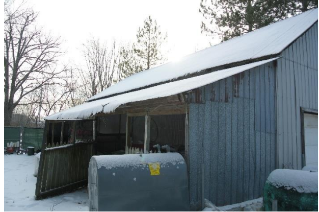
Image 11: View of the north addition to the one-and-a-half storey accessory building.
