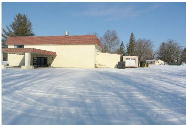
Image 7: View of the west and south elevations of the Clubhouse.
