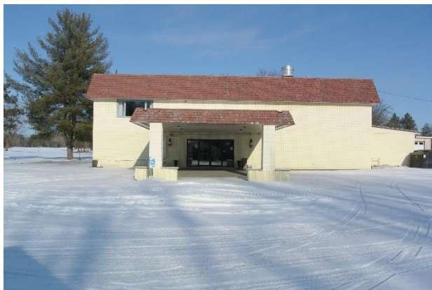
Image 6: View of the west elevation of the Clubhouse.
