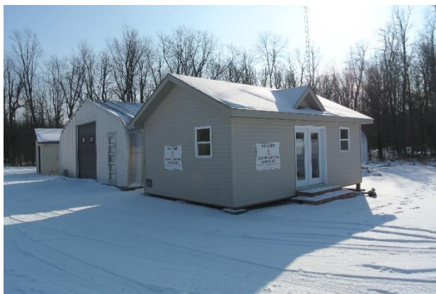
Image 9: View of the three accessory structures west of the Clubhouse, looking south.
