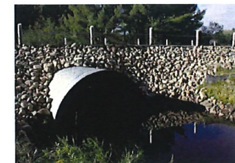
Black Bay Culvert, Petawawa, ON
