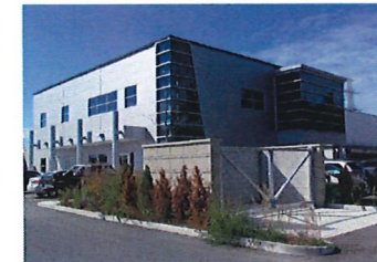
Cyr Distribution Centre, Ottawa, ON
