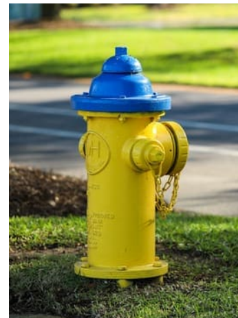
Figure 27: Proper Colour-coded Hydrant
