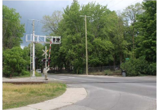
Figure 21: Railway Line running through Town
