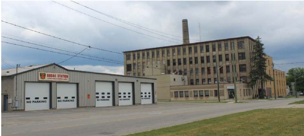
Figure 25: DNETV Fire Station 1 Located Within the Town of Perth
